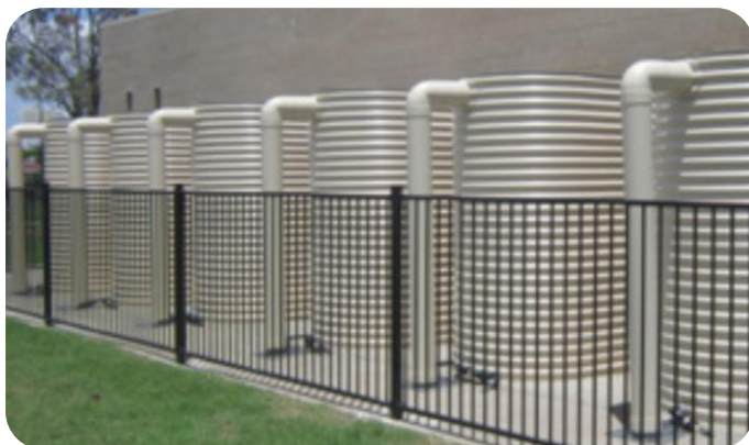
Ormeau Health Centre Multi-Bank Rainwater Tanks
