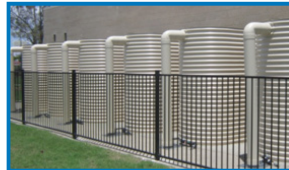
Ormeau Health Centre Multi-Bank Rainwater Tanks
